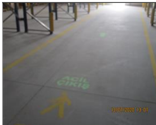
Photo of the inside of the main production hall Evacuation signs.JPG
