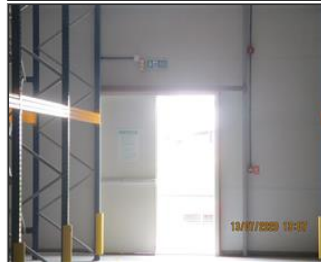
Photo of the inside of the main production hall Emergency exit door.JPG
